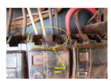
6.14 - There are white wires connected to breakers. Usually, this is indicative of improper wiring and it is safe practice to designate these wires with black or red tape at the breaker and the circuit end point to indicate the wire is hot and we recommend further review and correction by an electrician.
