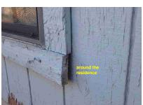
1.24 - Portions of the trim have peeling paint and we recommend it be serviced to prevent deterioration from the sun and moisture.
