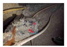
13.7 - An electrical connection has been incorrectly made outside of a junction box, which is a potential fire-hazard. We advise all such connections be made inside a junction box, in order to contain any arching or sparking within the box.
