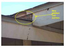
1.25 - The fascia boards are separating at the corners and we recommend these areas be sealed to prevent moisture damage.
