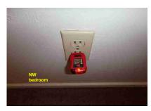
14.10 - An outlet is loose and needs to be re-secured to the wall.
