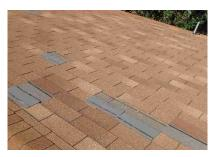
3.5 - Portions of the roof have exposed sheathing and we recommend immediate repairs.
