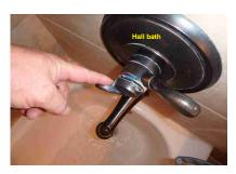
15.10 - The shower diverter valve in the tub/shower is defective, and we recommend it be serviced.
