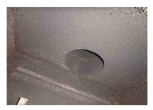
4.5 - The wood stove has buckled and warped due to over heating and we recommend it be further evaluated by a home heating specialist.
