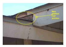
1.14 - The fascia boards are separating at the corners and we recommend these areas be sealed to prevent moisture damage.
