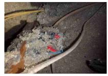
13.4 - An electrical connection has been incorrectly made outside of a junction box, which is a potential fire-hazard. We advise all such connections be made inside a junction box, in order to contain any arching or sparking within the box.
