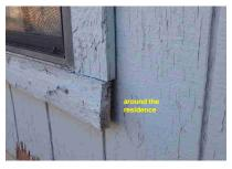
1.13 - Portions of the trim have peeling paint and we recommend it be serviced to prevent deterioration from the sun and moisture.
