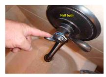
15.3 - The shower diverter valve in the tub/shower is defective, and we recommend it be serviced.
