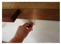
17.4 - An switch has a loose or broken cover and we recommend it be serviced.
