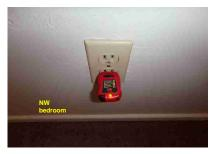
14.4 - An outlet is loose and needs to be re-secured to the wall.
