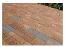
3.3 - Portions of the roof have exposed sheathing and we recommend immediate repairs.
